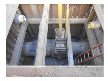
PLCS was tasked with designing, fabricating and installing a permanent repair system while at the same time, retaining the operational capability of the valve. The major challenge faced by the team of engineers and designers was devising a way to create a pressure-tight seal around the irregularlyshaped valve body. Confronted with the busiest shopping week of the year, it was imperative the project be completed swiftly to avoid disrupting the smooth running of the forthcoming celebrations.
