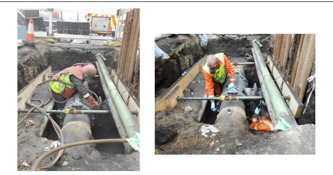
To avoid the weight of the heavy sealant (a quarter ton) slumping and distorting the mould, the teams created and fitted a strategically-placed framework of internal and external supports around the repair area.
