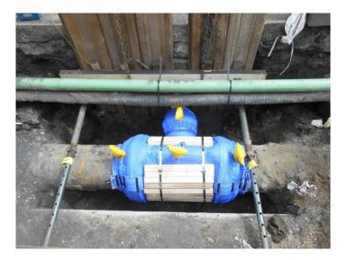
Being a hot summer's day, the team were faced with the challenge of mixing, pouring and pressurizing the encapsulant which had a work life of only 12-14 minutes due to the hot temperatures.
