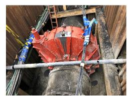
A follow up visit was necessary the next day to remove the spindle housing in order to retain the operational capability of the valve.
