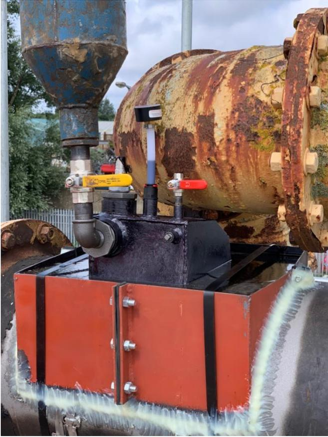
On day 3, the team returned to site. The shroud was applied, and the foot plate was fitted into place using metal bands, adhesive and encapsulate, ensuring that the heavily corroded fitting was secure.
