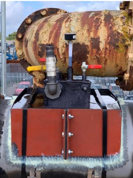
To repair the escape and combat the corrosion, PLCS Technical Manager, Mark Perry, Director Darren Billington and Team Leader Ross Fairley, set about making templates so that a metal mould could be fabricated to encapsulate the fitting.
